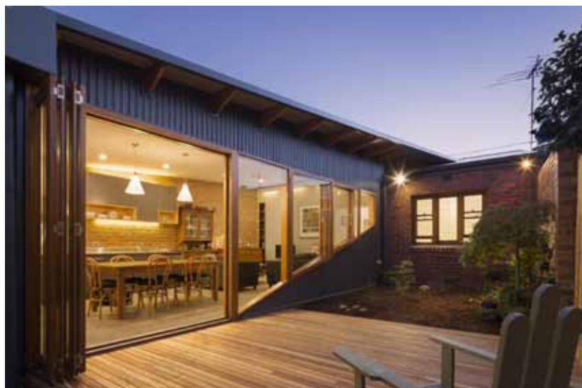
The steeply sloping roof profile forms a sunny second storey studio that maintains winter solar access to the southern neighbours.
